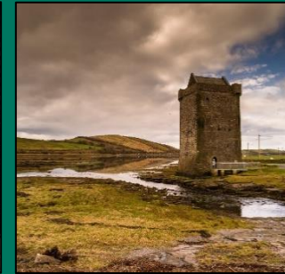
Rockfleet Castle, County Mayo, Ireland
