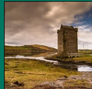
Rockfleet Castle, County Mayo, Ireland
